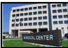
Memphis VA campus renovations, $44 million
